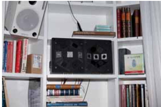
A terminal unit of the high-speed infrared communication system with transmit and receive sensors and emitters.
